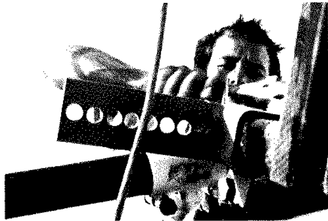
RETROFITTING the drive to the Paracclipse dish to accommodate the IQ-160 drive system. McLaughlin is a hard worker.
